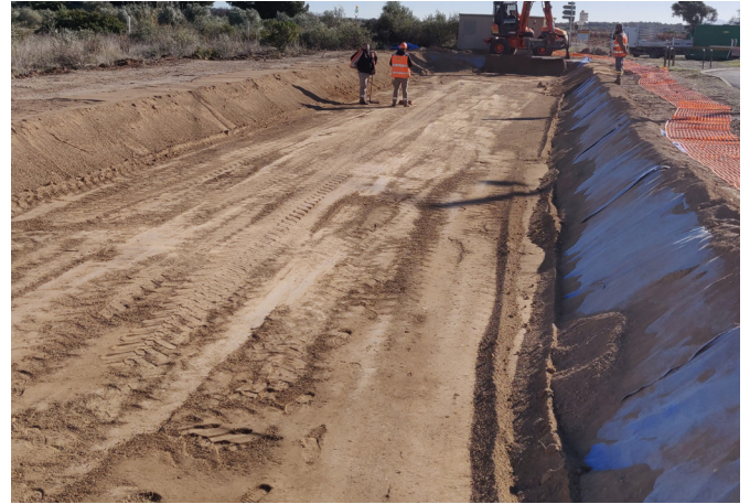
Figure 5: Covering the bottom and slopes with permeable soil
