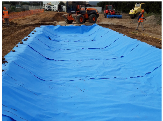
Figure 1: Laying aquatextile strips on the bottom and slopes of the structure, with soil blocks used for ballasting at the top
