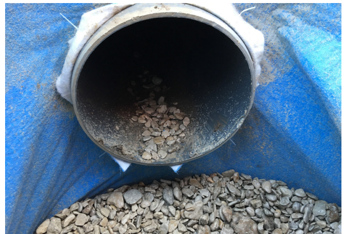
Figure 3: Pipe passes through aquatextile in the cut-out
