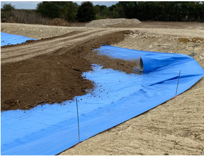
Figure 6: Completing the installation by covering the aquatextile with permeable topsoil in the infiltration basin
