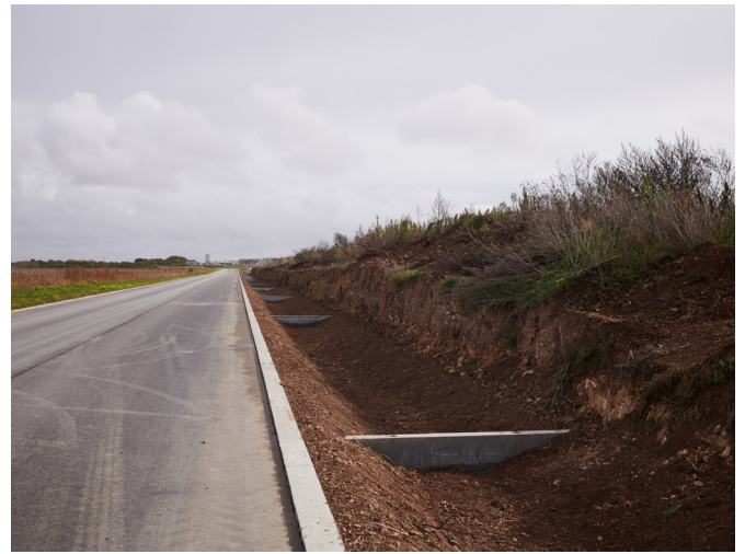
Figure 7: Covering the aquatextile with permeable topsoil
