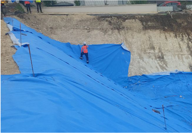
Figure 4: Staking the strips in place at the top of the slope
