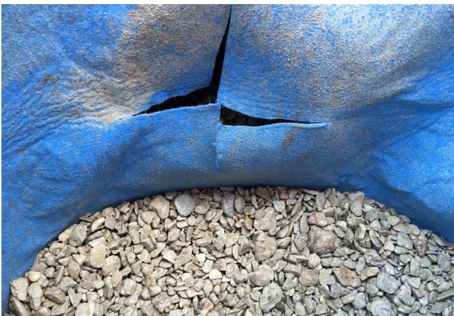
Figure 2: Cross-cutting of aquatextile for pipe passage
