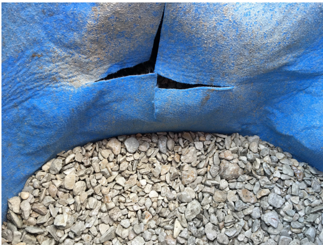
Figure 1: Cross-cutting of aquatextile for pipe passage
