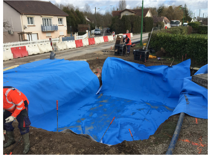
Figure 4: Installing aquatextile strips at the bottom and sides
