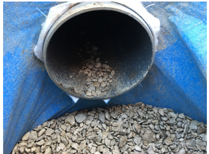
Figure 2: Pipe passes through aquatextile in the cut-out
