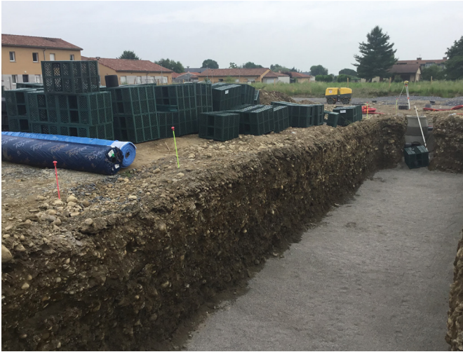
Figure 3: Surface preparation (e.g., draining layer)
