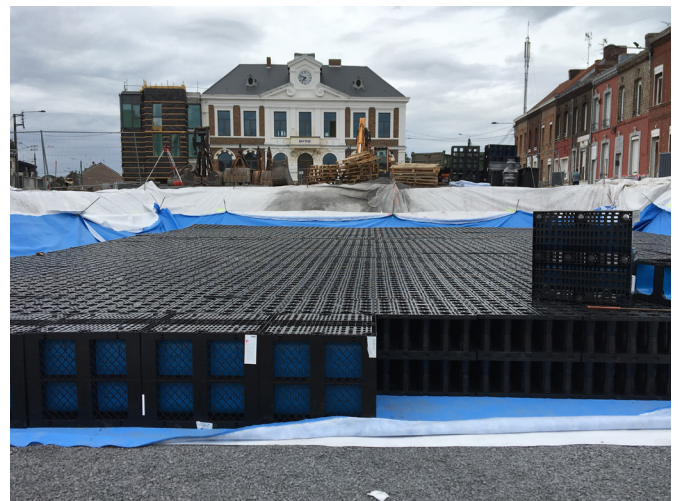
Figure 4: Installing aquatextile strips at the bottom and sides
