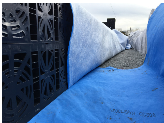
Figure 6: Raising strips on the tank
