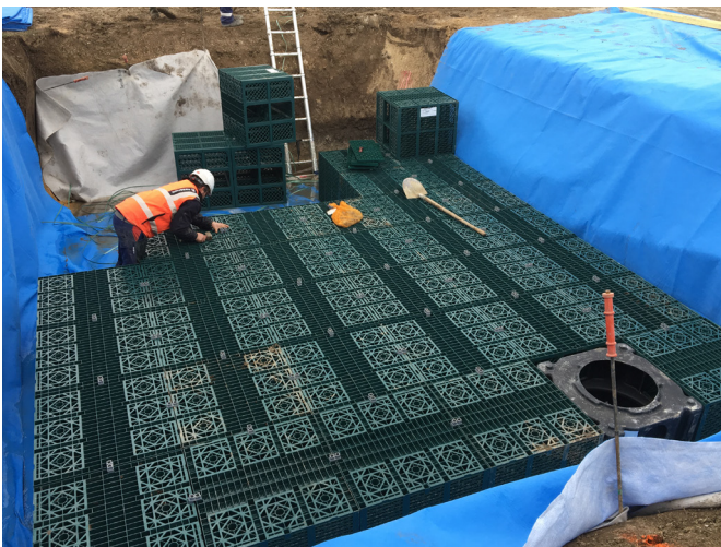
Figure 5: Crate installation
