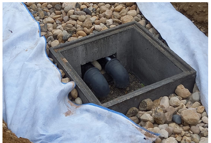
Figure 6: Covering the top of the granular mass with at least 30 cm of aquatextile, pending installation of a separation geotextile
