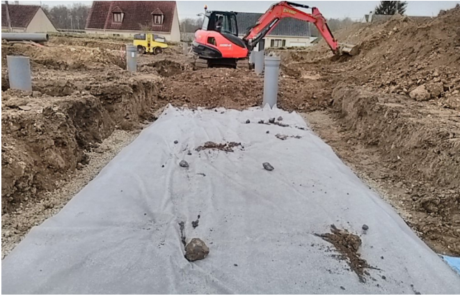
Figure 7: Covering the buried structure with a separation geotextile, at the end of backfilling the trench with granular material
