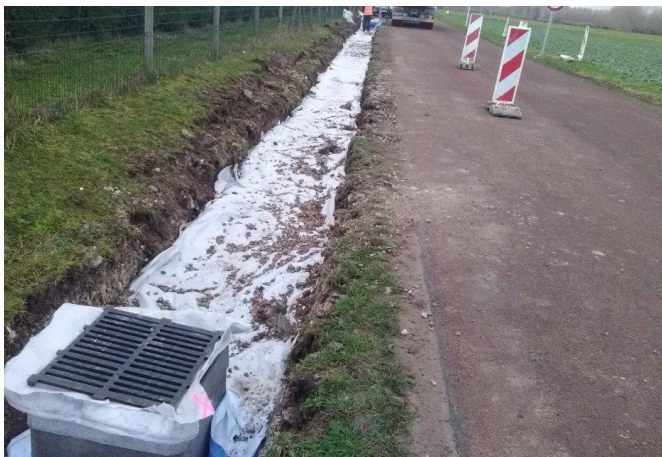
Figure 3: Covering the granular mass by the extra length of the aquatextile left on hold
