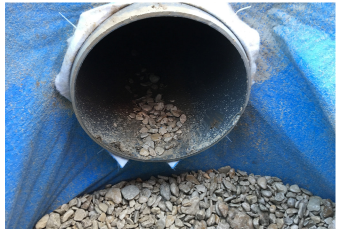
Figure 2: Pipe passes through aquatextile in the cut-out
