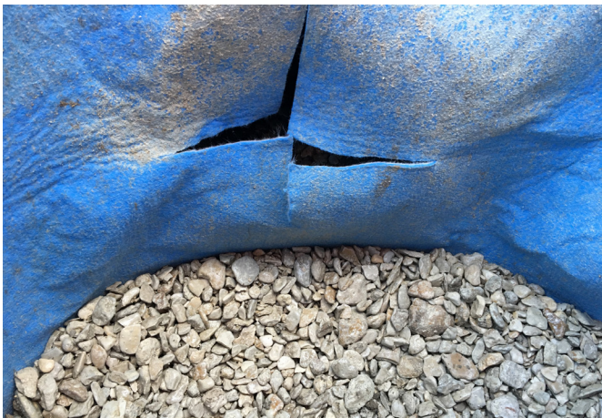
Figure 1: Cross-cutting of aquatextile for pipe passage
