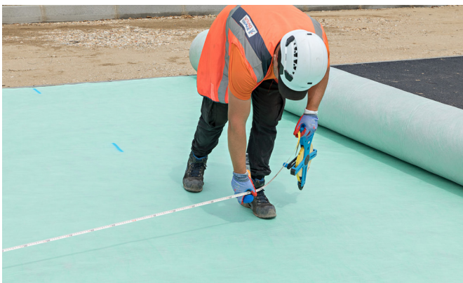
Figure 2: Measuring and cutting strips, if necessary
