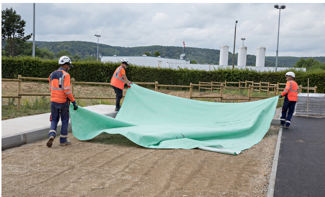
Figure 3: Installing the aquatextile with a 30 cm overlap on horizontal surfaces
