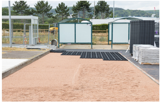
Figure 5: Grading the surface and installing the permeable coating (e.g., honeycomb slabs)
