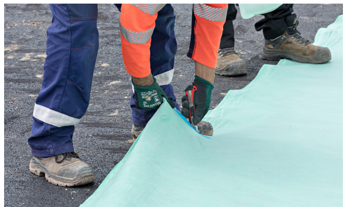
Figure 1: Subgrade preparation
