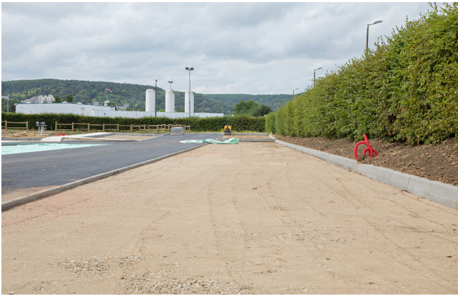
Figure 5: Grading the surface and installing the permeable coating (e.g., honeycomb slabs)
