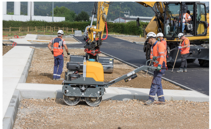
Figure 1: Subgrade preparation
