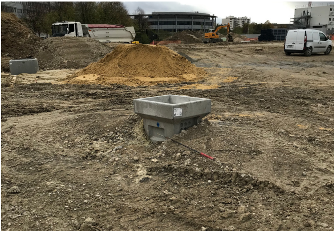
Figure 2: Injection well with a decanter to collect rainwater from an impermeable surface and inject it into the reservoir structure. The decanter reduces the amount of solid particles entering the buried structure
