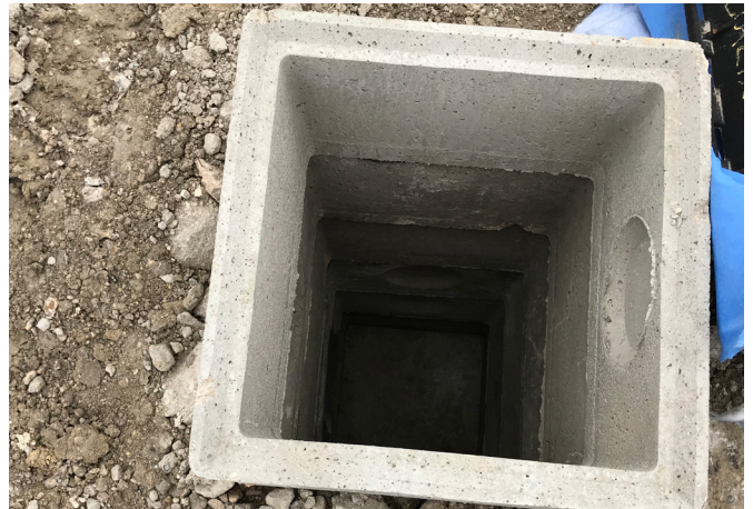
Figure 2: Injection well with a decanter to collect rainwater from an impermeable surface and inject it into the reservoir structure. The decanter reduces the amount of solid particles entering the buried structure
