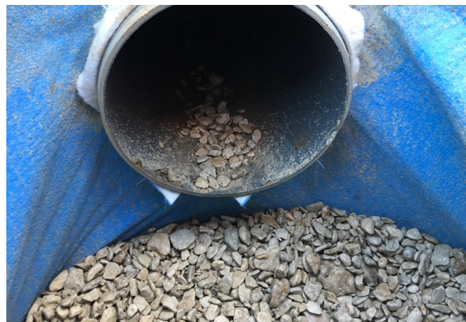
Figure 2: Pipe passes through aquatextile in the cut-out
