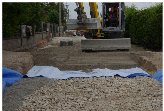
Figure 6: Backfill placed over the reservoir structure wrapped with OSMORIA Geoclean aquatextile
