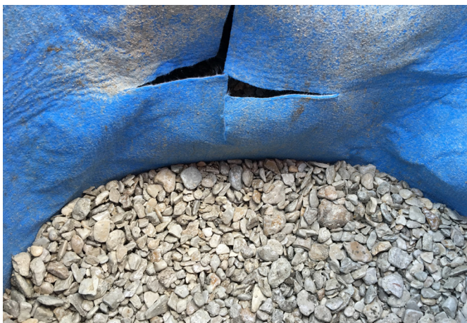
Figure 1: Cross-cutting of aquatextile for pipe passage
