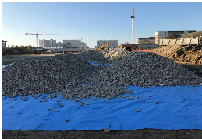
Figure 3: Ballasting of the OSMORIA Geoclean aquatextile and installation of the granular reservoir structure
