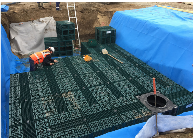
Figure 5: Pose des caissons
